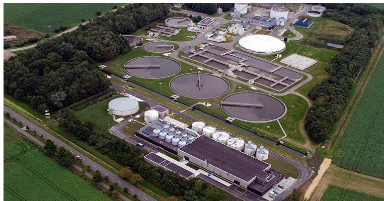
Figure 4: The Schoonebeek water treatment facility.
