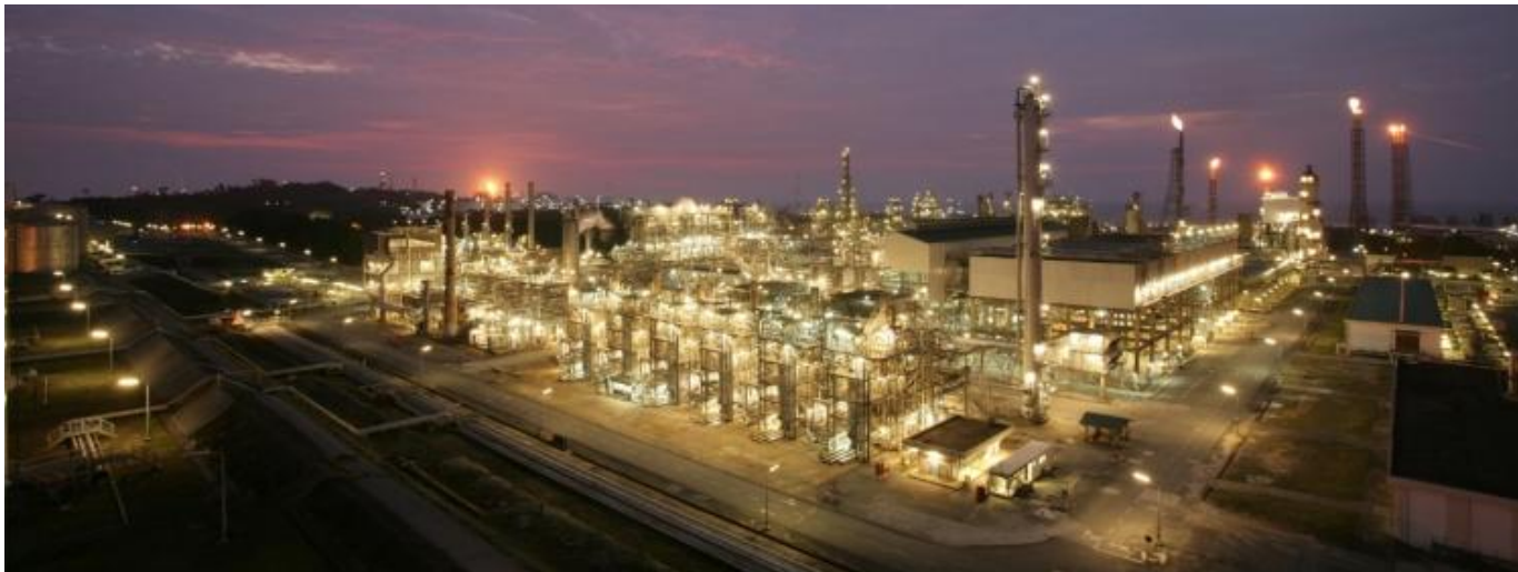
Figure 5: The Pearl Gas to Liquids complex.
